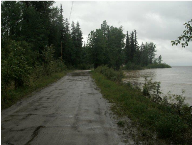
Moberly Lake shoreline and overland flood impacts (2011)
