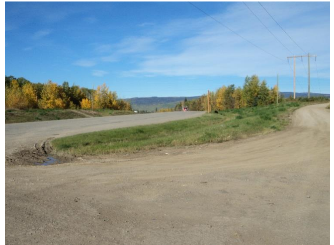
Fig#2: Access looking west along Hart Highway (97S) towards Chetwynd
