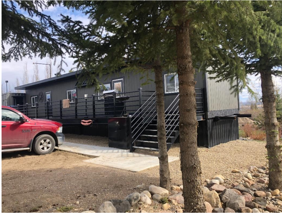
Image 1. The existing office located near the front parcel line and the south interior side parcel line as detailed in Schedule B.
