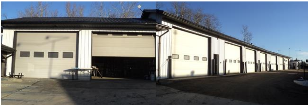
Image 2. The existing shop located near the north interior side parcel line as detailed in Schedule B.
