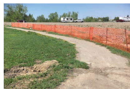
Existing Dawson Trail looking towards 8th Street. Upgrades to address erosion issues and damage would be required.
