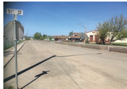
Looking west along 49th Ave.
