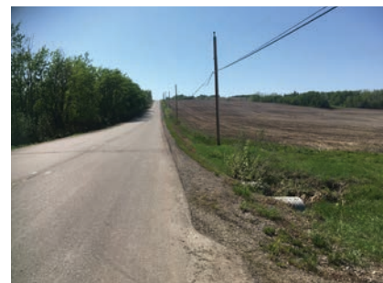
Creek crossing on 244 Rd looking west towards 271 Rd.
