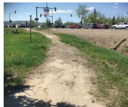
Existing Dawson Trail looking towards 8th Street. Upgrades could be completed to improve the trail and develop a visible, accessible trailhead.
