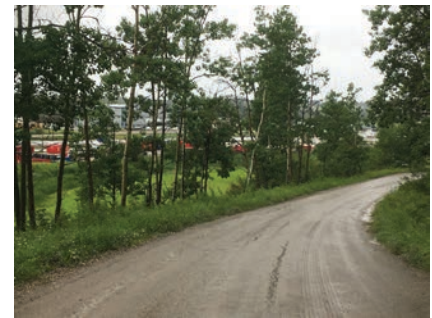
Looking southwest down Rimrock Dr with significant grades on adjacent slopes.
