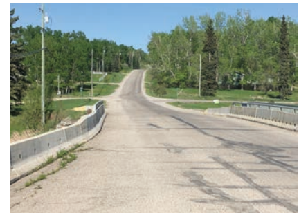
Looking north towards Rimrock Dr from the existing Fish Creek bridge. The proposed pedestrian crossing could occur at Rimrock Dr with development of a new pedestrian bridge at Fish Creek adjacent to the vehicle bridge.
