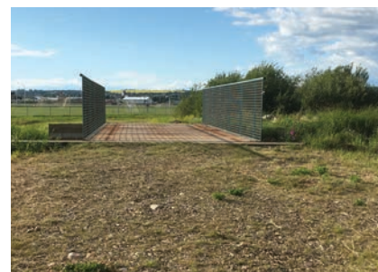
Existing bridge over the creek near the Encana Events Centre.
