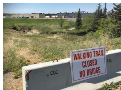
Location of washed out bridge.
