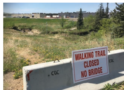
Location of washed out bridge.
