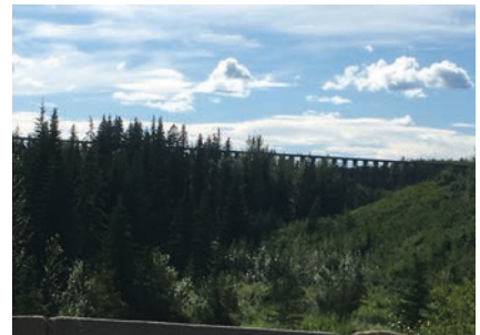
View toward CN trestle looking west from Rolla Rd.
