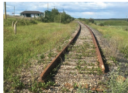
CN Rail corridor looking north from Hwy 2 near McNabb Recreational Park.
