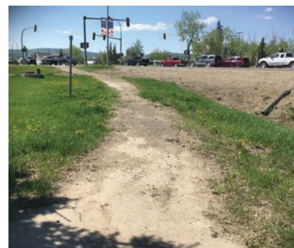
Existing Dawson Trail looking towards 8th Street. Upgrades could be completed to improve the trail and develop a visible, accessible trailhead.
