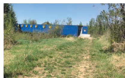
Rotary Seacan Bridge and natural surface trail.
