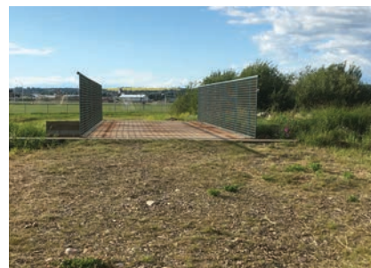
Existing bridge over the creek near Encana Events Centre.
