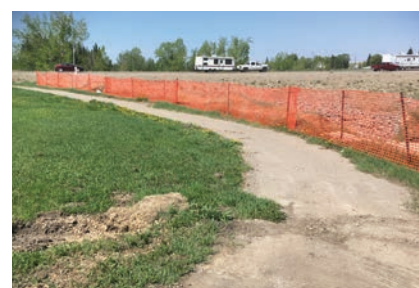
Existing Dawson Trail looking towards 8th Street. Upgrades to address erosion issues and damage would be required.
