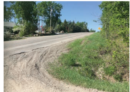
Looking north up 269 Rd from Kapchinski Rd.
