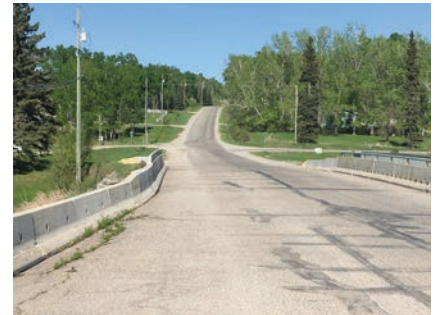
Looking up Sunnyside Drive from Fish Creek.
