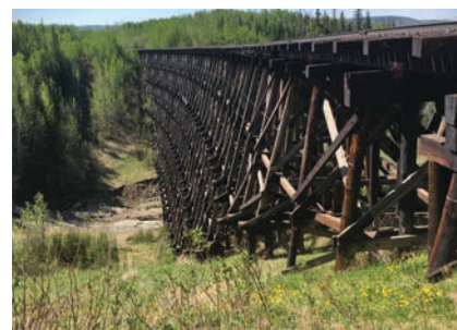
Existing railway trestle.
