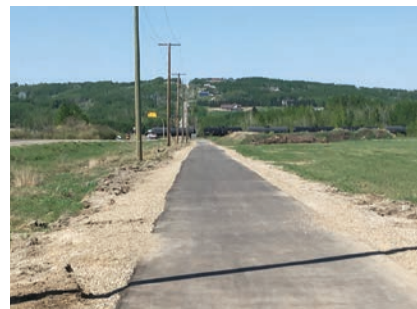
West Bypass Trail looking north towards CN Rail tracks.
