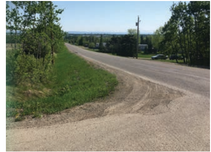
Corner of Kapchinski Rd/269 Rd looking south.
