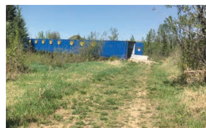
Rotary Seacan Bridge and natural surface trail.
