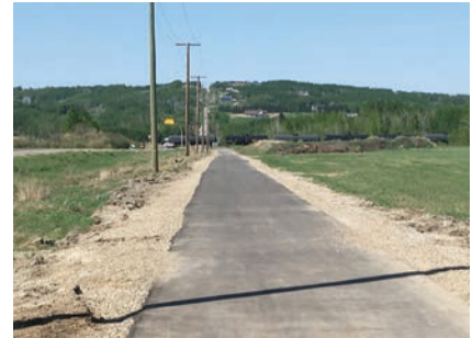
West Bypass Trail looking north towards CN Rail tracks.
