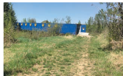
Rotary Seacan Bridge and natural surface trail
