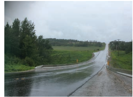
Looking north up 271 Road at the Fish Creek bridge.
