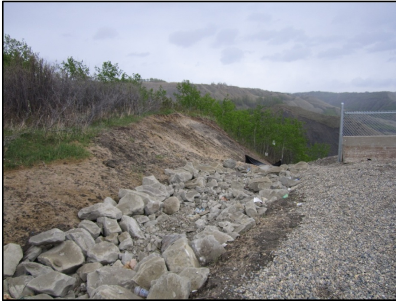
Slide 2.2b: Rip rap installed in the drainage ditch to the left of the viewing area
