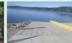
Improved boat ramp
