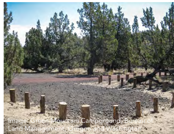
Example of wood bollards used to define the extents of a Vehicle Area where it may not be obvious based on vegetation.
