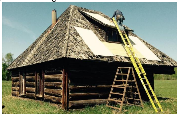
Ken Boon temporarily stabilizes the roof to prevent further leaks.
