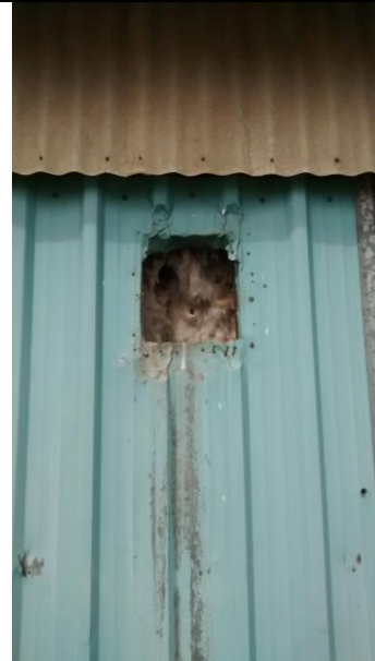
E Wall Open Penetration (1)
