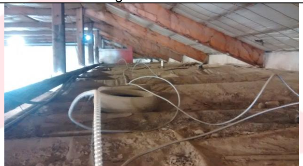
Roof of Kitchen Area
