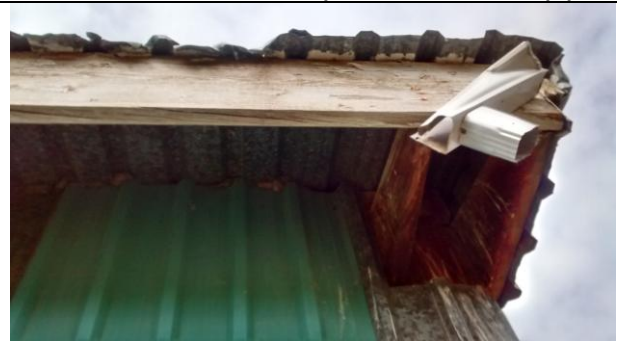
NE Corner – Evidence of Gutter System
