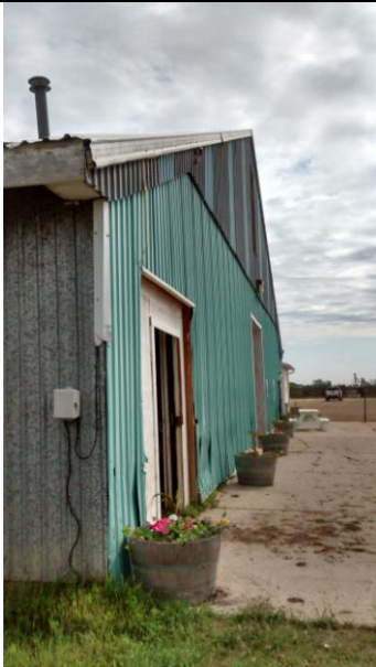
S Roof Line
