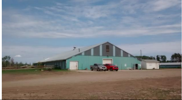
SW View of Arena
