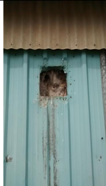
E Wall Open Penetration (1)
