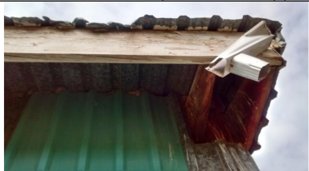
NE Corner – Evidence of Gutter System
