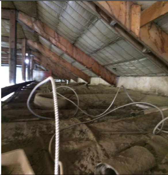
Roof Above Kitchen
