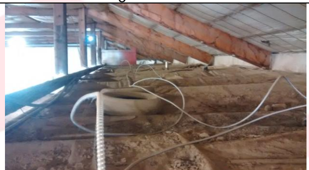
Roof of Kitchen Area
