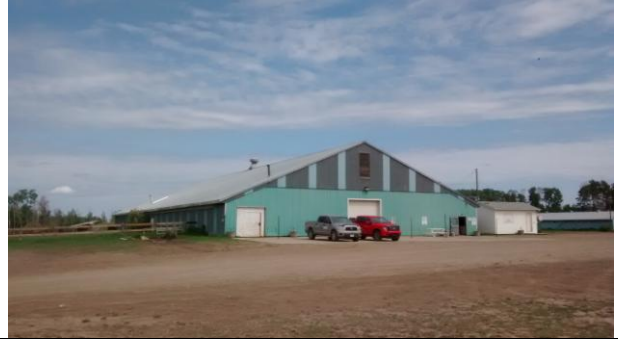
SW View of Arena
