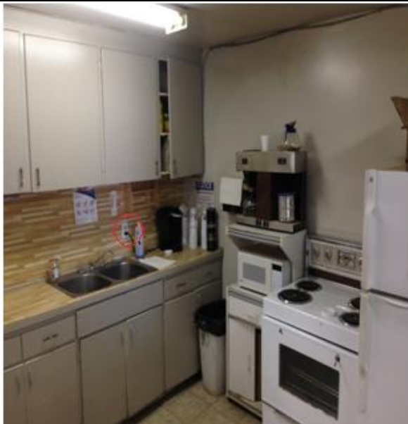
Receptical Near Sink
