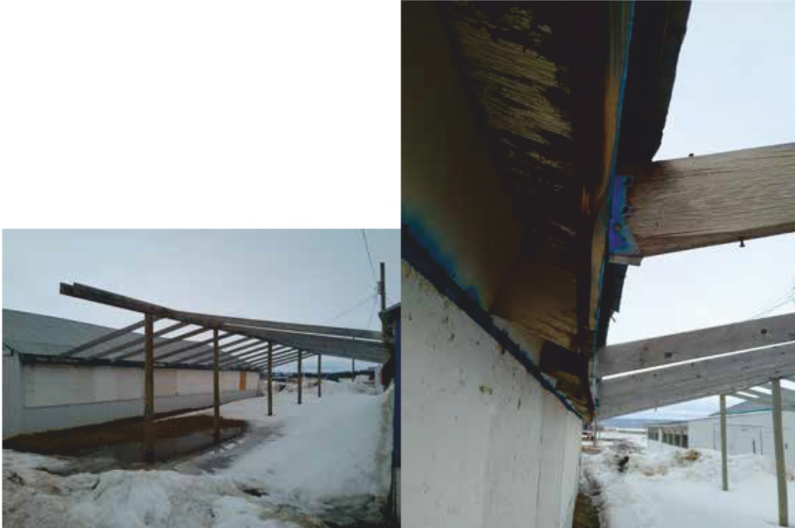
"Tent" between Stables 7.7 and 7.6. Framing Arrangement to Stable 7.7 Eave
