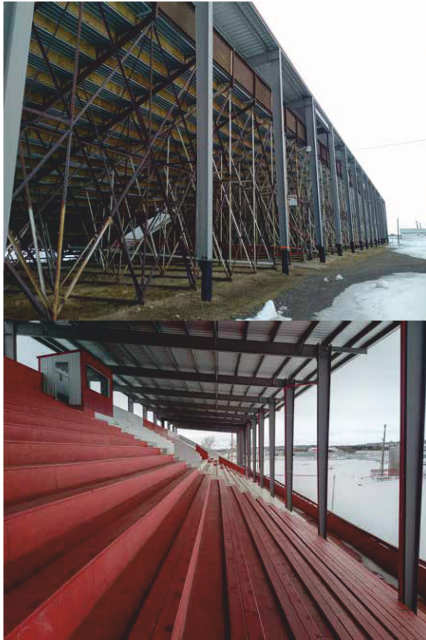
Grandstands Overall Spring 2018
