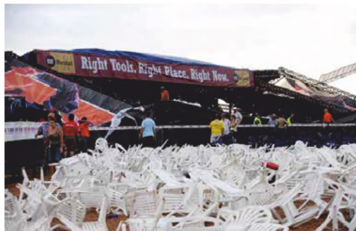
Big Valley Alberta Stage Collapse 2009. 1 killed, 75 Injuries
