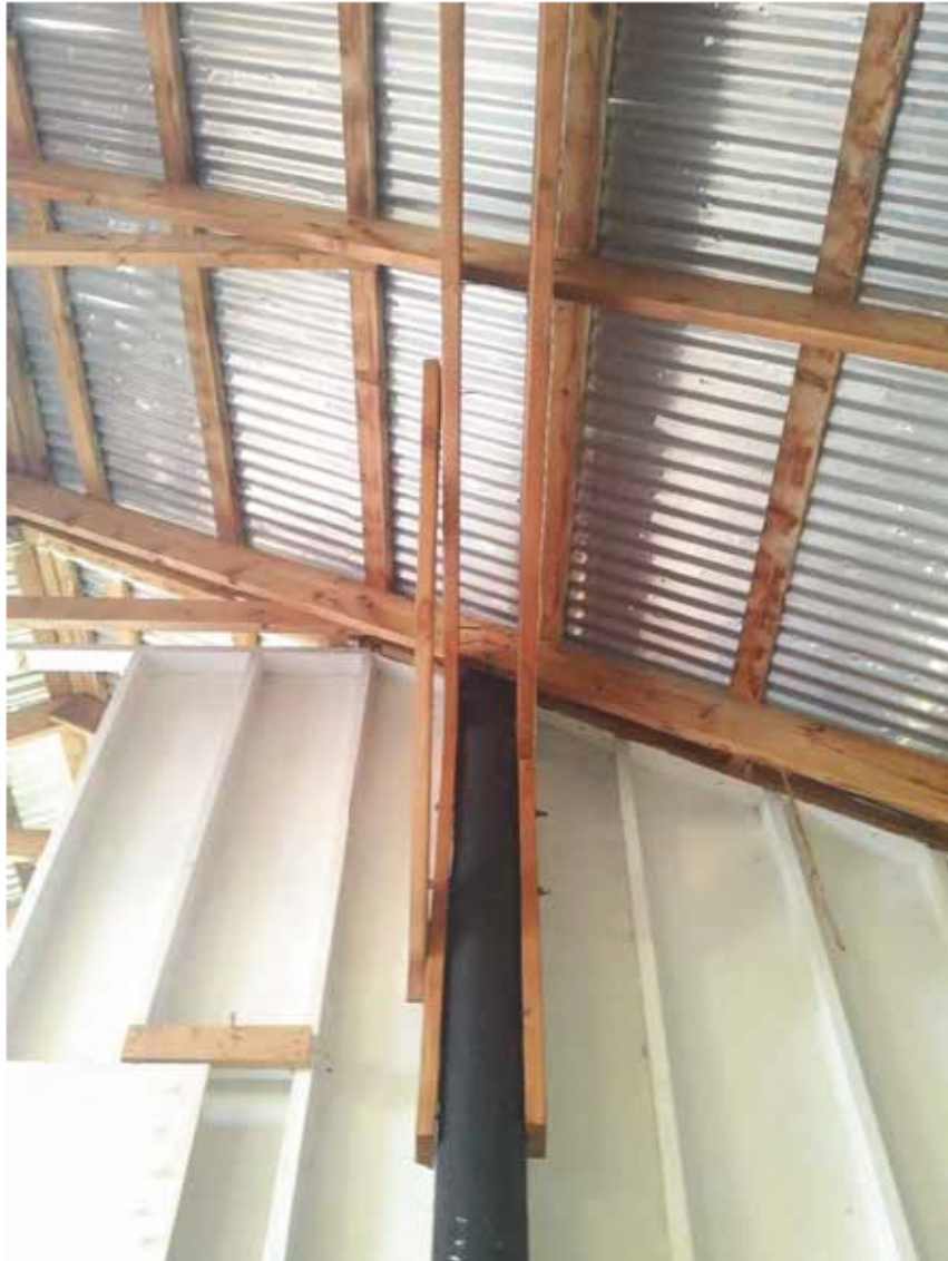
Single Ply Load Bearing "Beams" Spanning 15'-0"
