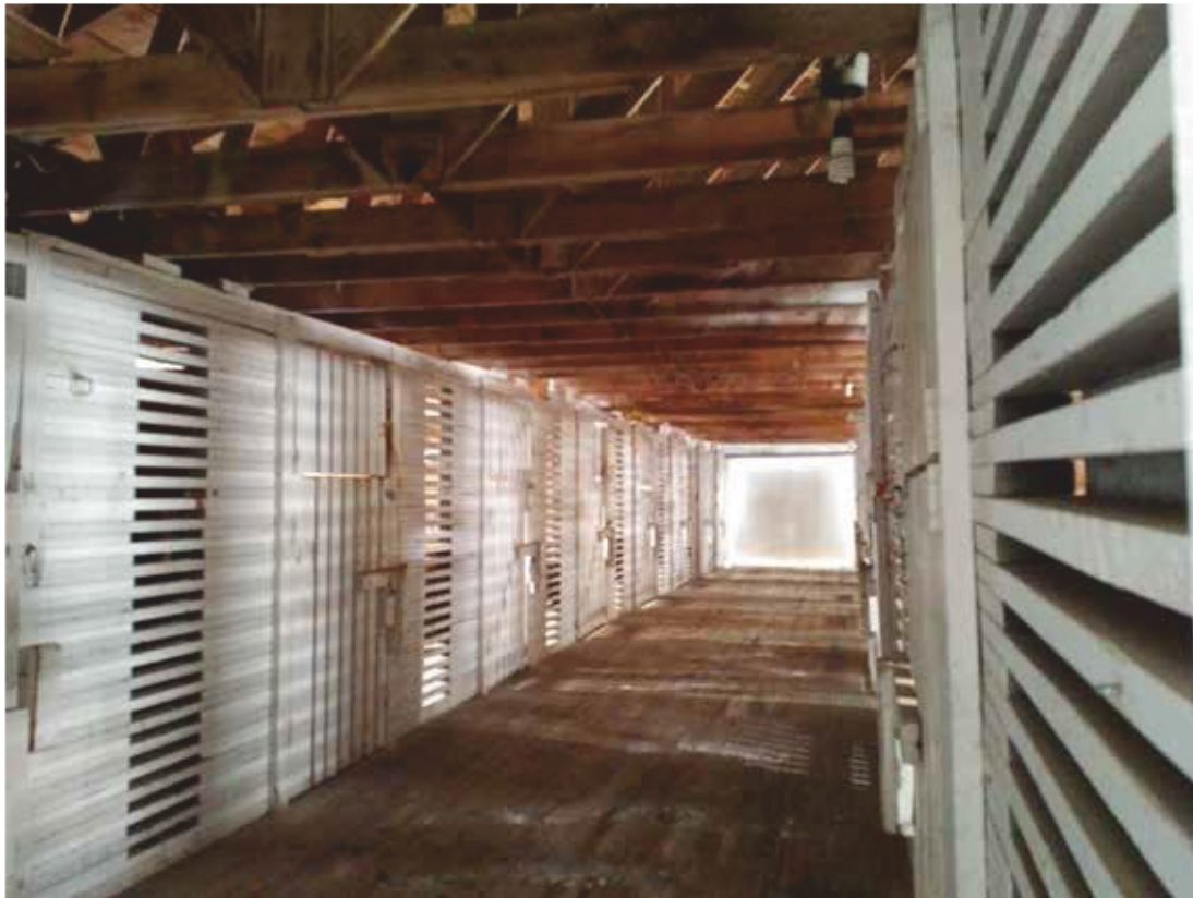
Stable 7.1, Interior State, Painted – No Structural Improvement Noted.
