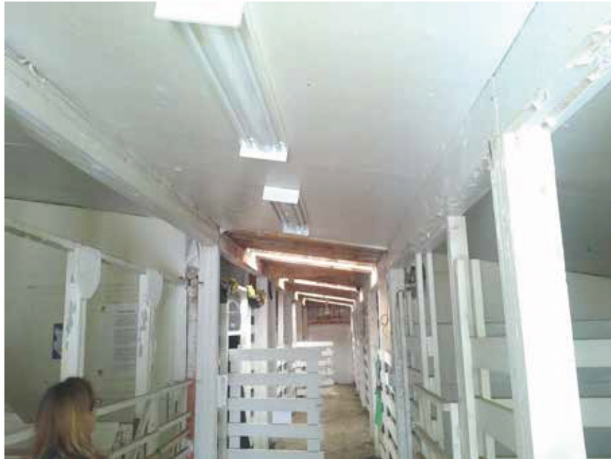
South Lean To Interior
