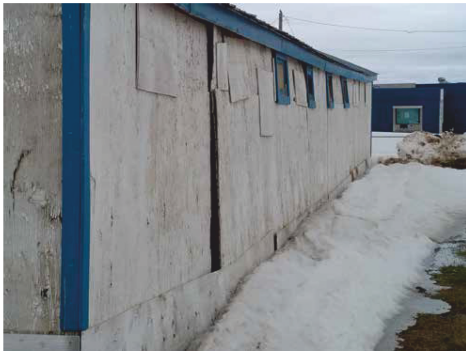
Exterior State, Typical
