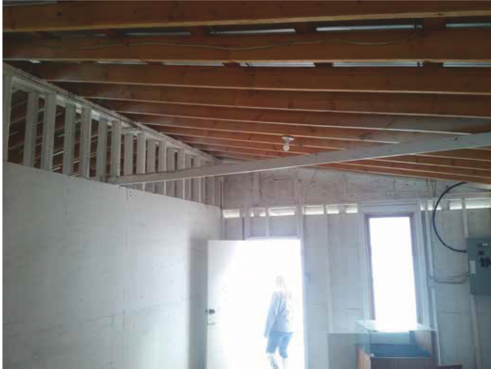
Building 'D' Interior Showing Framing
