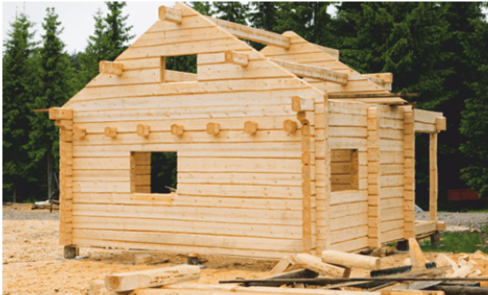
Typical Milled Lumber Log Framing Arrangements
