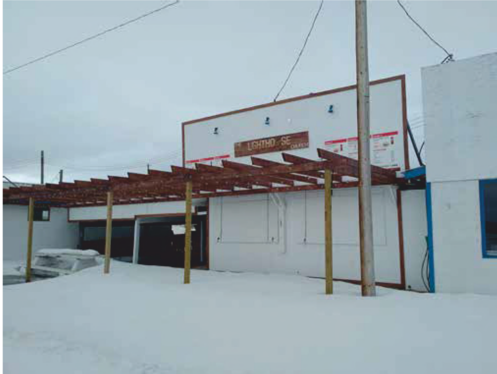
Building 'C' Overall
