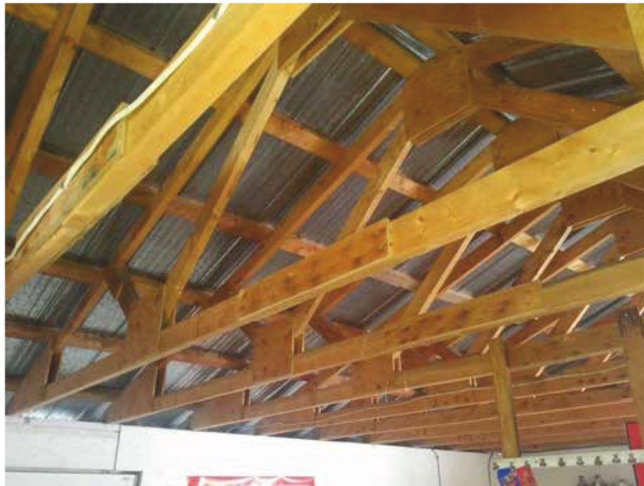
Job Site Manufactured Trusses Overall Arrangements
