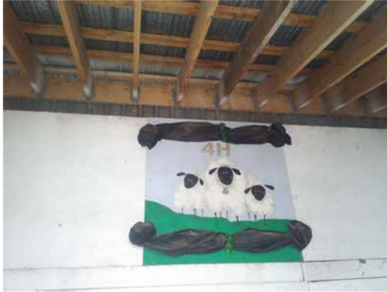
South Lean To Addition Connection to Centre Building
