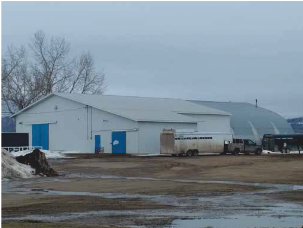
Riding Arena with Reconstructed Portion at Left, Arch Roof Structure at Right
