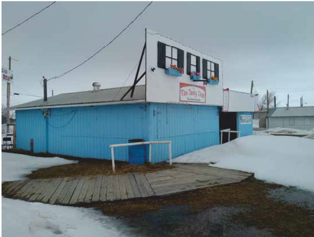
Structure as Reviewed, Kitchen at Left, Covered Seating at Right
