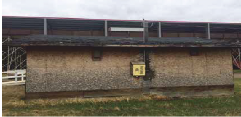
South Elevation, April 2016, Prior to Repainting
