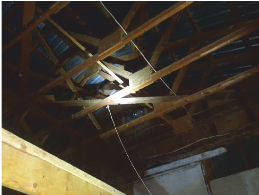
Centre Portion – Heavy Horse Barn Jobsite Fabricated Trusses
