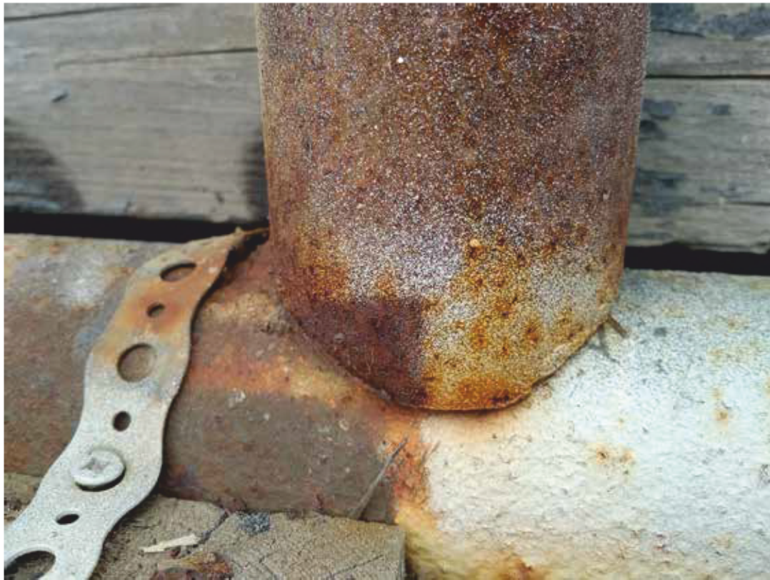
Weld Joint with Minimal Bead
