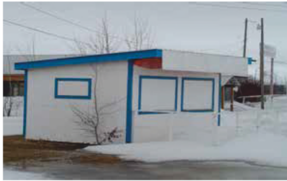
Building Overall, Showing Limited Decay on Lower Sheathing
