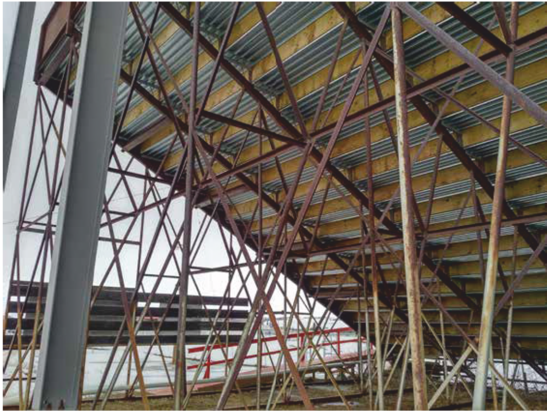
Condition of Steelwork, Western End
