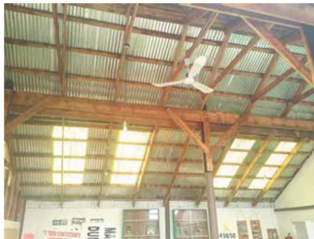
Roof Assembly General Arrangement with Undersized Elements
