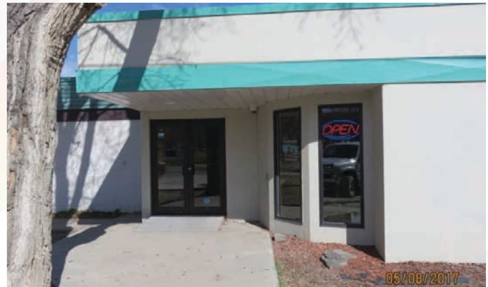
The front entrance is not well marked.
