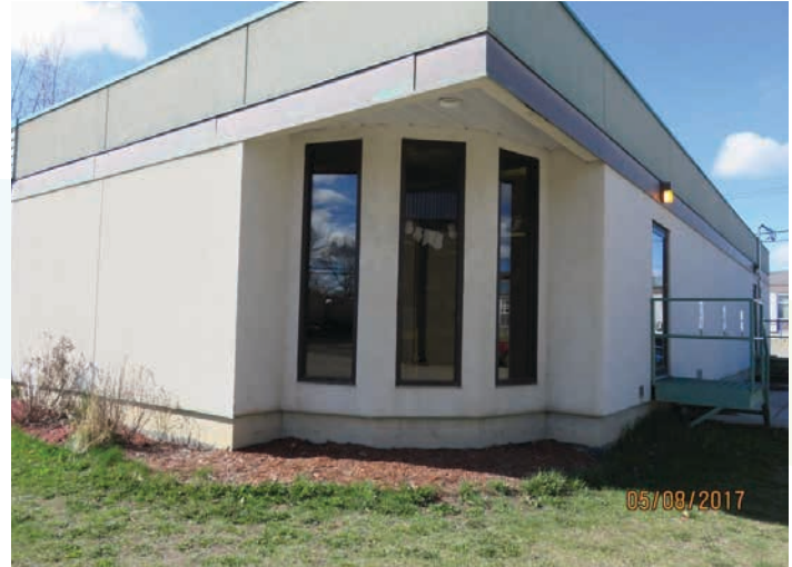
Back of building—minimal landscaping.
