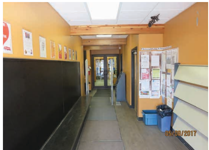
Entry is narrow and constricted by furnishings.
