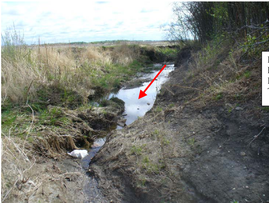
Photo 8 – Rolla Creek just below #217 Rd. looking downstream. Erosion is ongoing upstream of site shown in Photo 7 despite rock gabion works.
