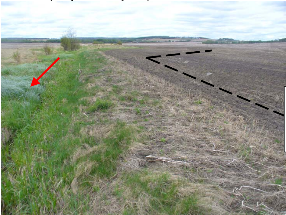
Photo 6 – Rolla Creek immediately upstream of #215 Rd showing current limited channel capacity due to sediment deposition. Containment dyke would be located along north/left bank /right side in the photo
