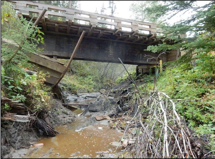
DS elevation. Hanging crib wall.
