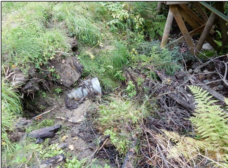
Culvert outlet. Flow directed to piers of DS bridge.
