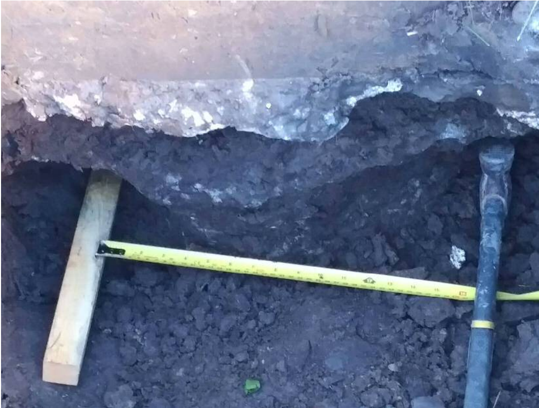
Piling Size Measurement
