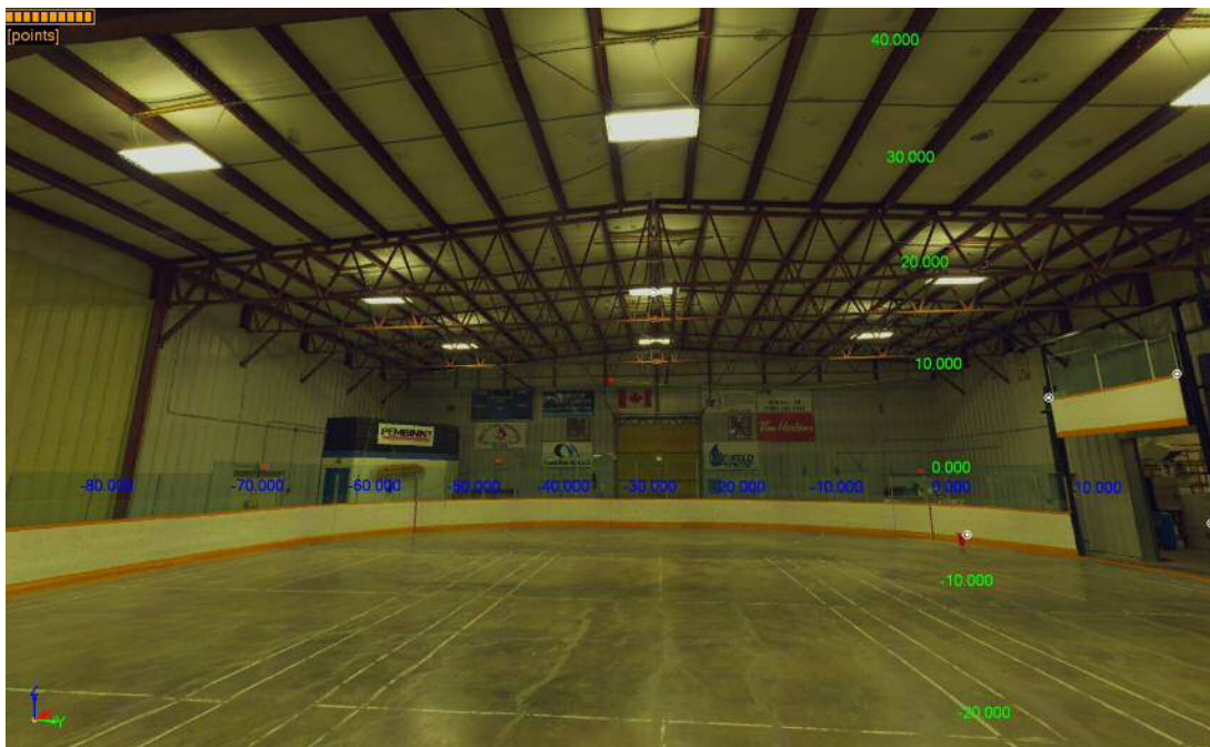
Photo View of Building Interior
