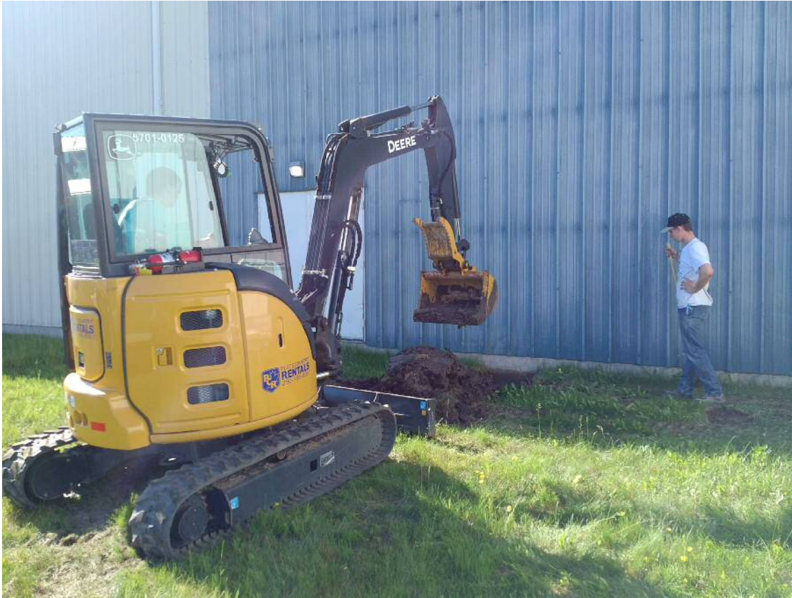
Excavation of Piling at Grids "A" and "9"
