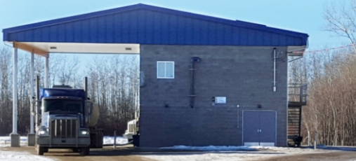
Newly completed Truck sewage waste receiving facility located on 273 Road south of the Alaska Highway.
