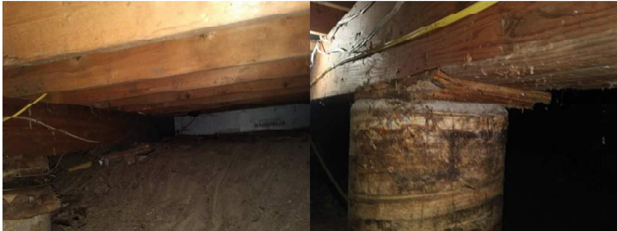
Beam End in Contact with Grade, Plywood Shims Under Beam Deteriorating
