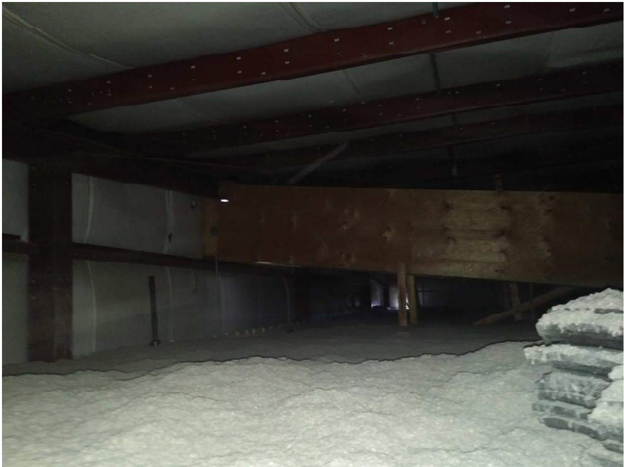
Attic Over Second Floor. Steelwork in near Original Condition
