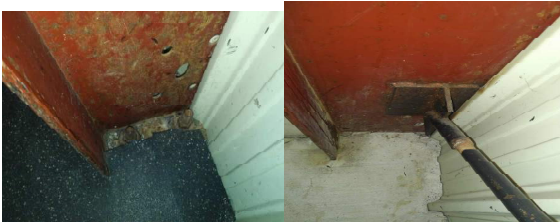
Exposed Anchor Bolts (Left ) and Relocated, Welded Brace (Right)
