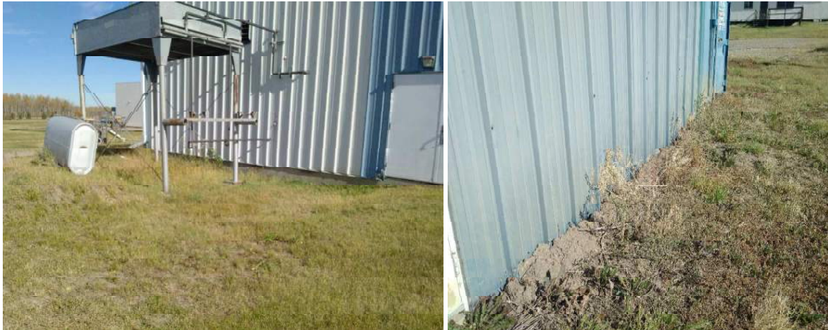
West Wall Grades Slope towards Building. Grade at SE Corner is Over Cladding
