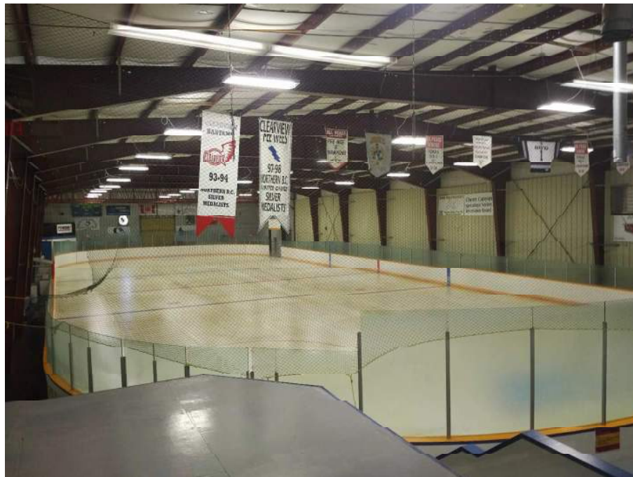
1975 Frame (Butler) Building
