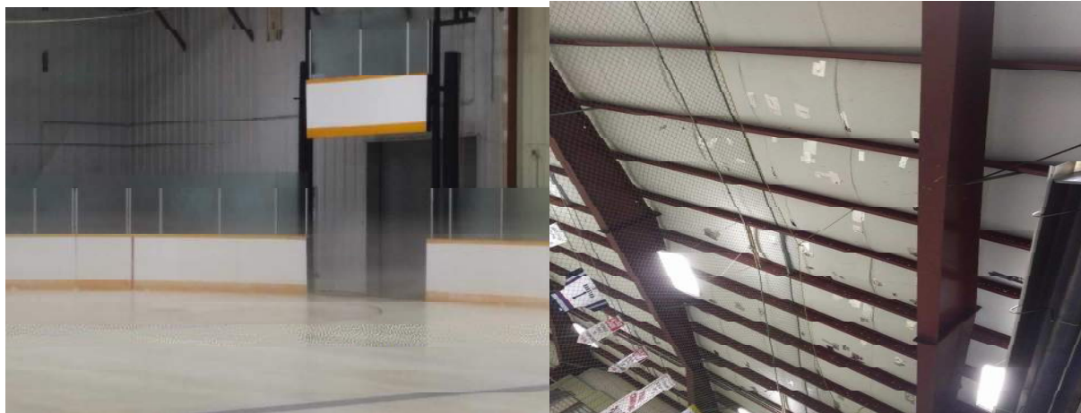
Fog and Condensation (Left) and Vapour Barrier Patchwork (Right)
