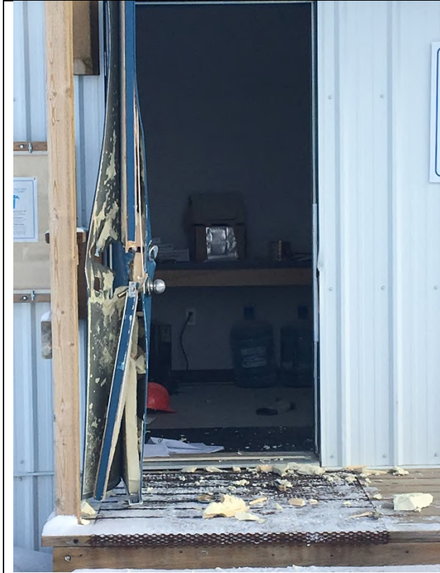
Photo 1: Entrance door into Goodlow Transfer Station attendant shack.
