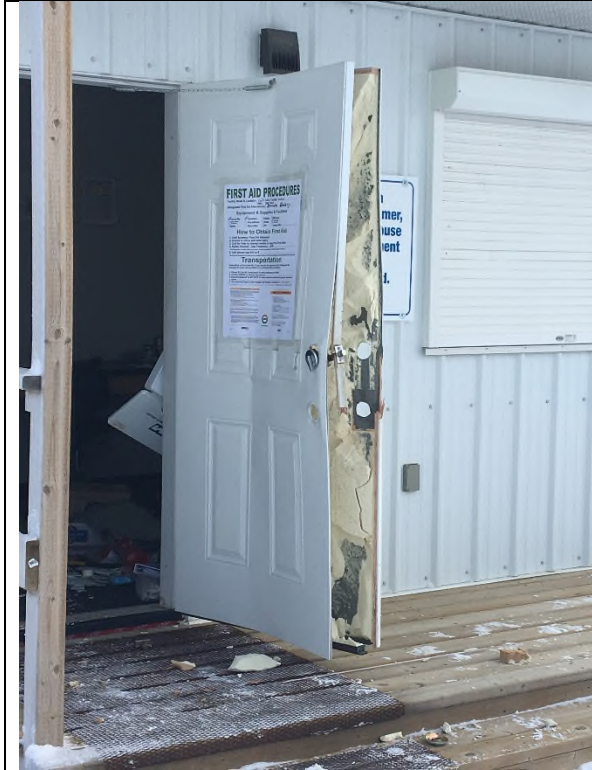
Photo 6: Entranceway door to Cecil Lake Transfer Station.
