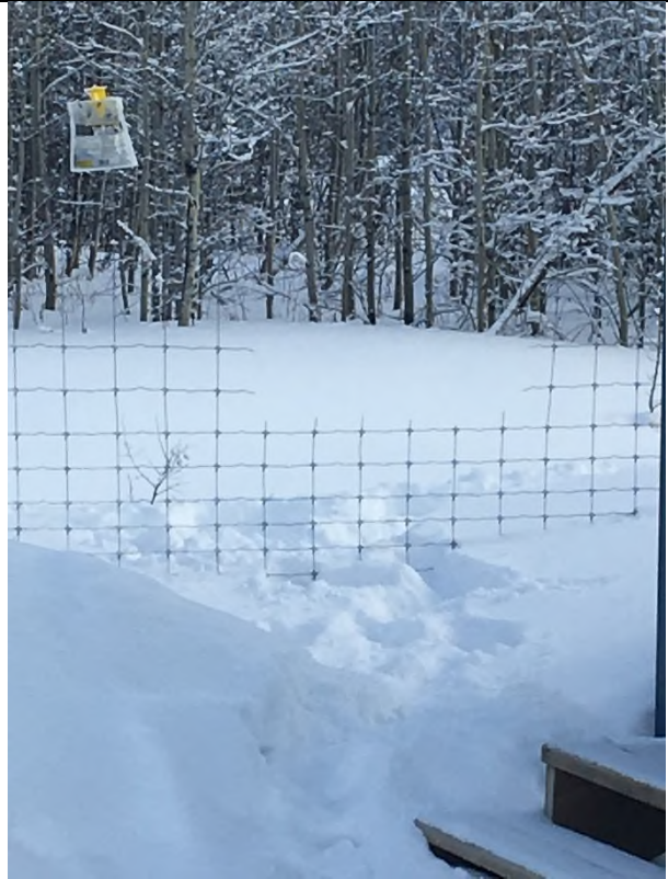
Photo 2: Fencing damage Goodlow Transfer Station.
