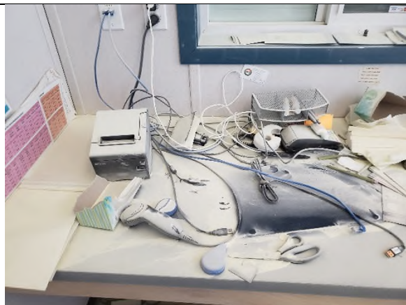
Photo 4: Electronics at Goodlow Transfer Station covered in Fire Extinguisher material.
