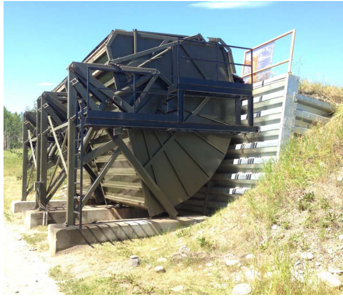
Transtor units and retaining Wall
