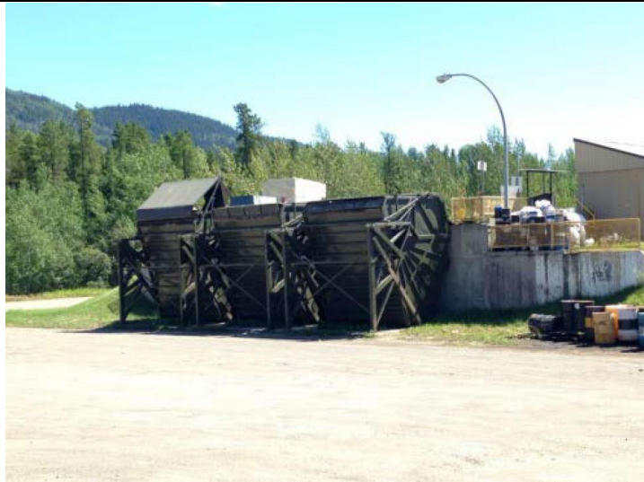
Figure 2 Transtor Bins - Rear View (Tumbler Ridge)
